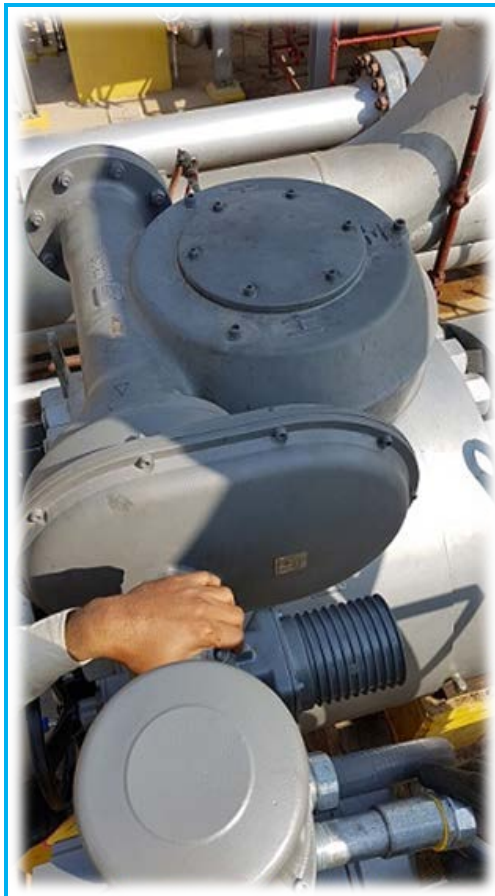
Figures 15 & 16 show newly deployed electrical actuators at SWID facilities
