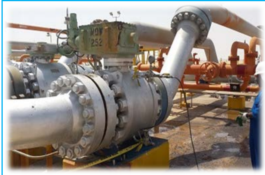
Figure 7: Ball valve's cavity venting/drainage & flushing application
