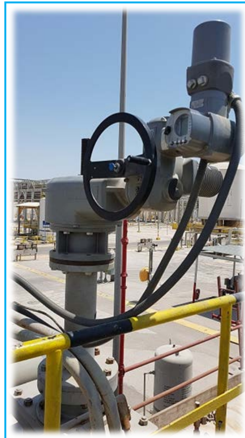
Figures 15 & 16 show newly deployed electrical actuators at SWID facilities
